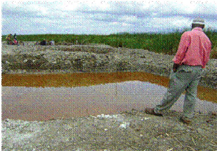
Figure 16. A community member appreciates the ponds constructed at Jipe through the project
