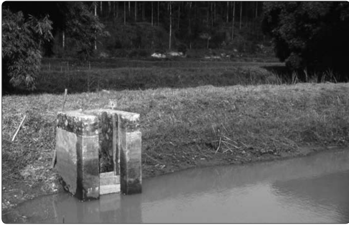
Figure 2.2-8. Although more expensive to construct, monks are sometimes used instead of standpipes. In this example, some of the upper boards have been removed to lower the water level in the pond.
