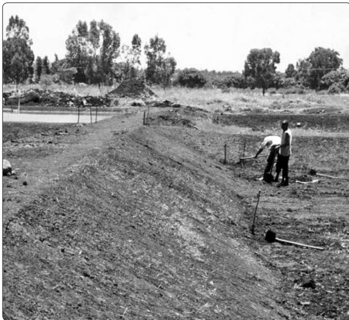
Figure 2.1-2. A well designed pond allows for a water depth of about 1 metre and has embankments (dykes) with inside slopes of 2 to 1 or greater, depending on soil type.
