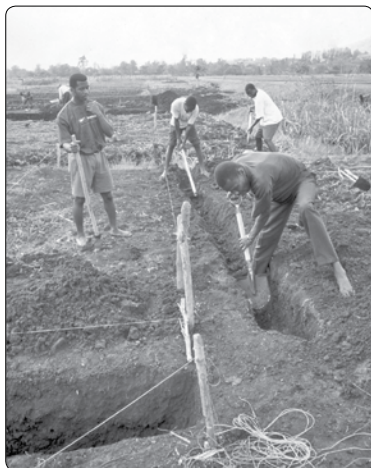
Figure 2.2-3. This area has been pegged out and core trench digging has begun. The core will be packed with soil containing not less than 30% clay before dyke construction begins.
