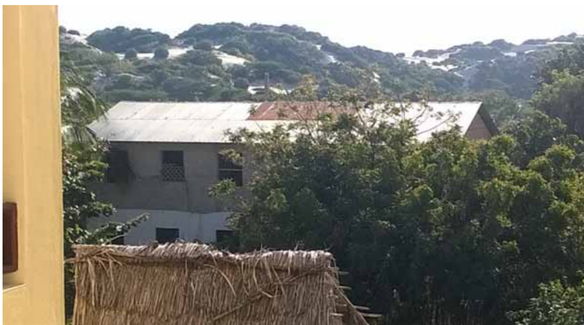
Plate 31: Settlement encroachment onto the Lamu Island sand dunes (Photo: Onywere, Oct. 2015)
