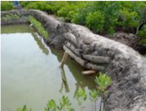
Figure 2. A pond at Majaoni showing stand pipe for draining the pond and overflow pipes to relieve the pond of extra water at spring high tides and increase water exchange in the culture ponds.
