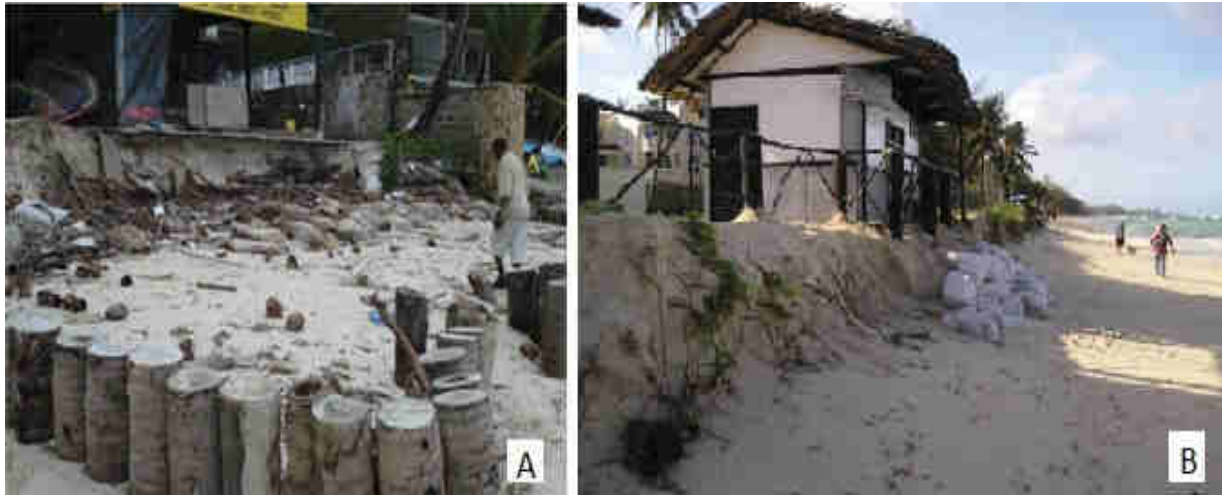
Plate 8.6 Sea front buildings threatened by erosion at Bamburi (Source: Shaghude et al. 2015; Arthurton, 2003)
