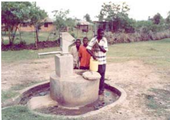
Picture 9. Broken Obuso well with open access
