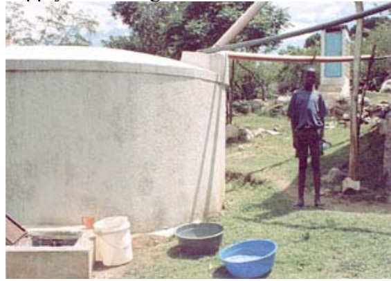
Picture 18. Ferro cement RWH tank built by SANA
