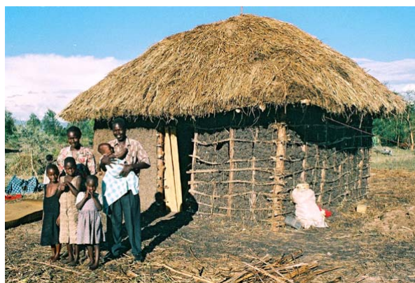
Picture 4. Traditional home under construction
