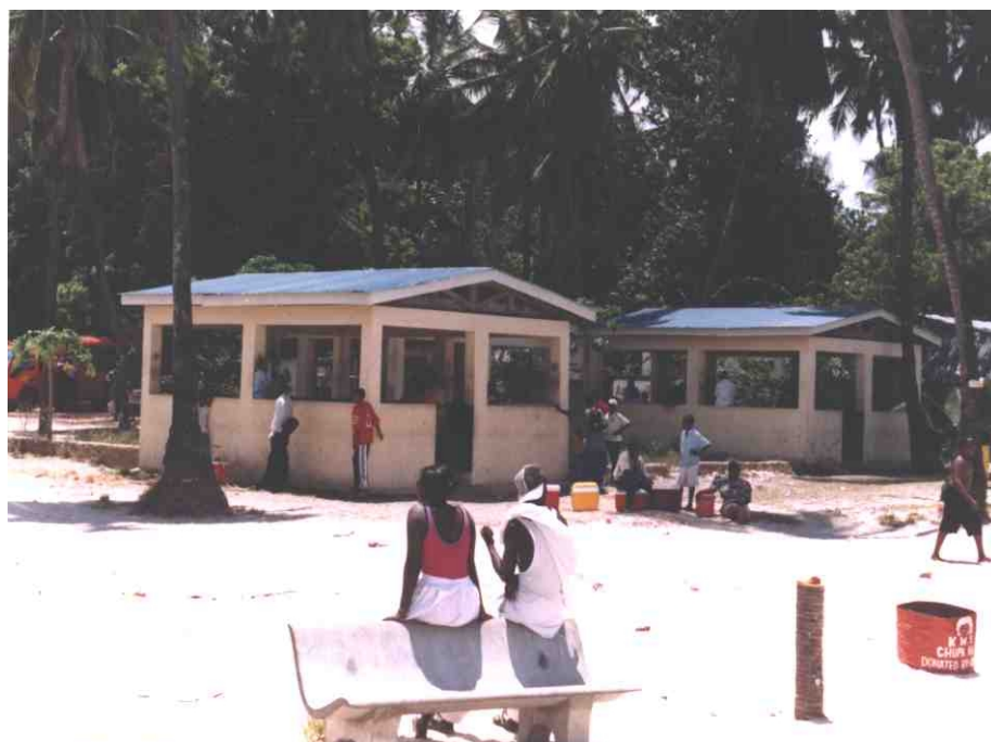
Photo 5: Jomo Kenyatta Public Beach construction
