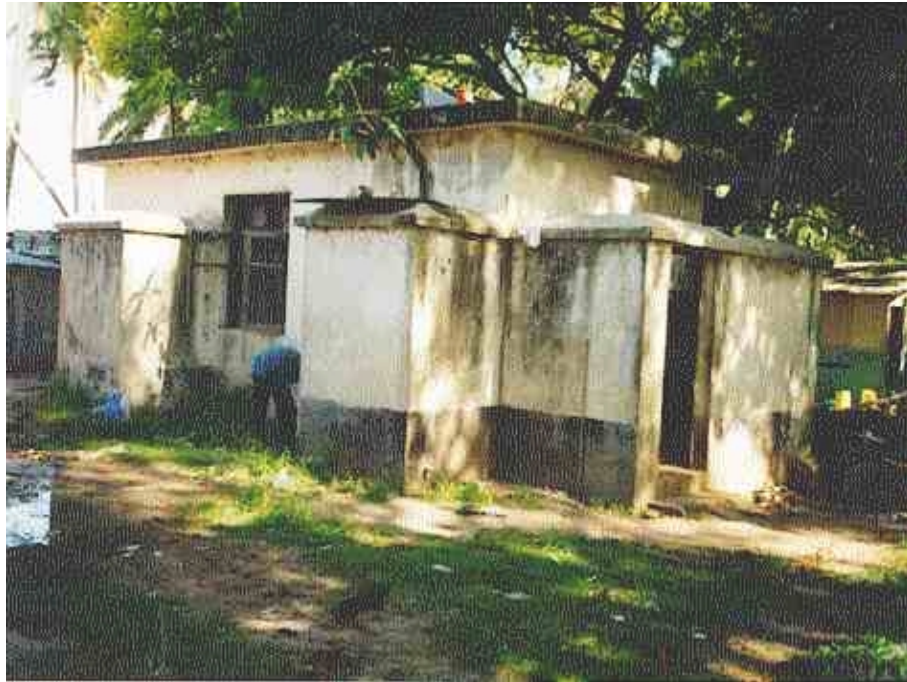
Photo 6: Jomo Kenyatta Public Beach construction
