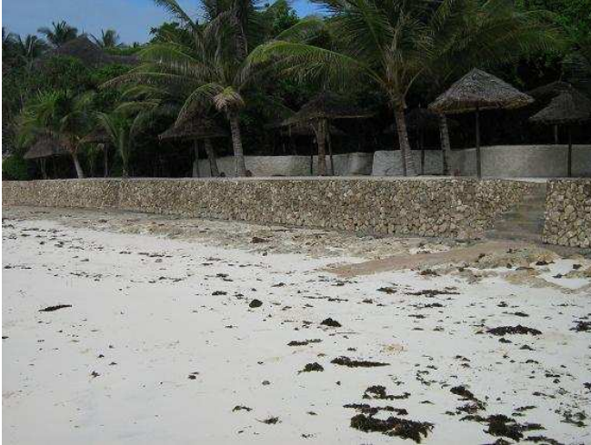
Figure 6-4: Leopard Beach Hotel in April. During the following months the entire beach will erode. Photo: CF57
