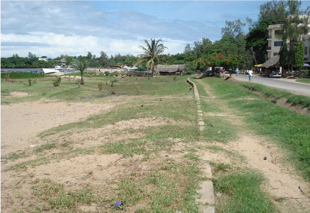
Figure 31: Section 5, old seawall. Photo: CF57
