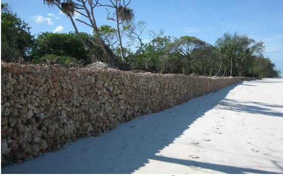
Figure 7-14: Vertical seawall in Diani Beach. Photo: CF57
