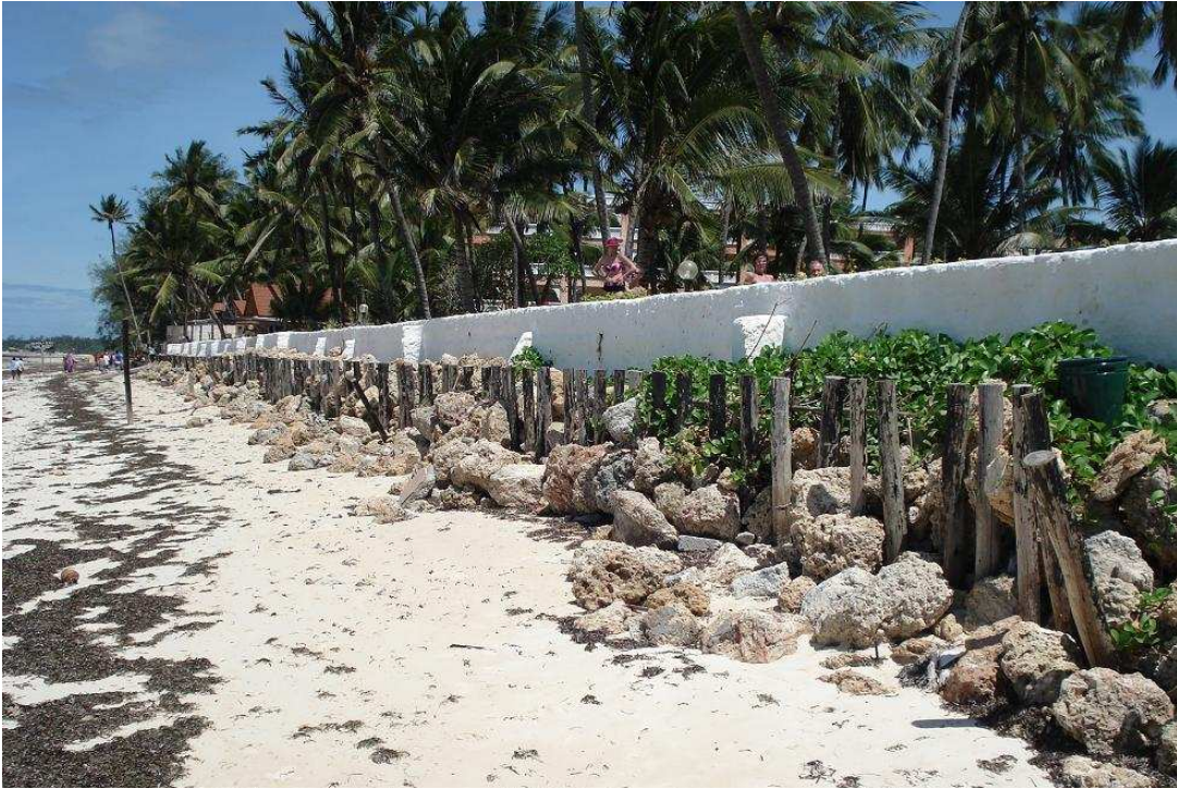
Figure 26: Section 2, seawall at Sun N Sand Beach Resort. Photo: CF57
