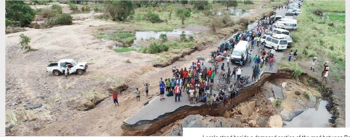
Locals stand beside a damaged section of the road between Beira and Chimoio in Nhamatanda district, central Mozambique, on March 19, 2019, after the area was hit by Cyclone Idai. Source: © National Institute of Disaster Management, Mozambique.
