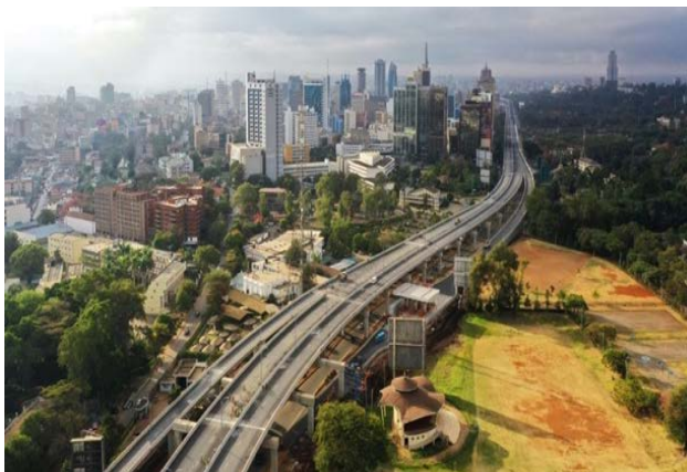
(b) The Nairobi Expressway
