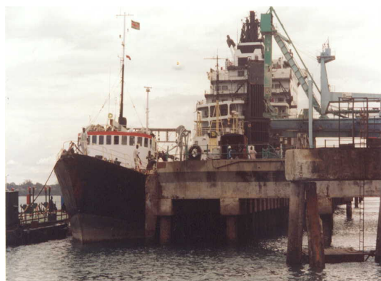
Figure 5a: Port facility
