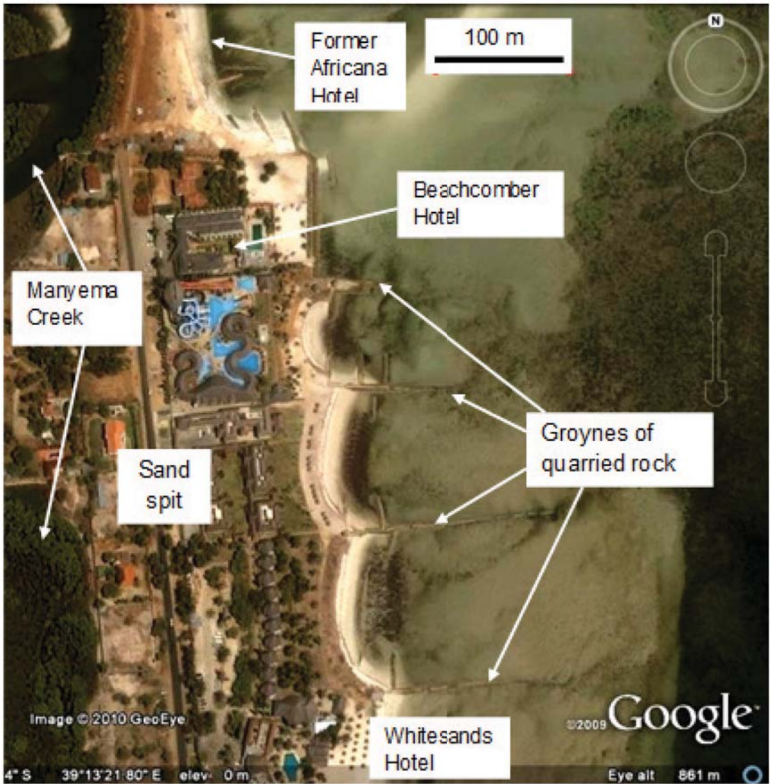
Fig. 49. Groynes of quarried limestone installed along the seaward side of the sand spit between the Beachcomber and Whitesands hotels on the Kunduchi shore. Note the scalloped form of beaches between the groynes. Image 20 December, 2003 ©2010 GeoEye.
