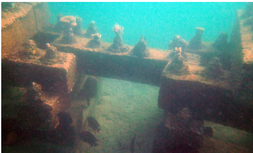
Plate 2. Artificial concrete structures with view of fish concentrations after one year Operational cost of community-based restoration project
