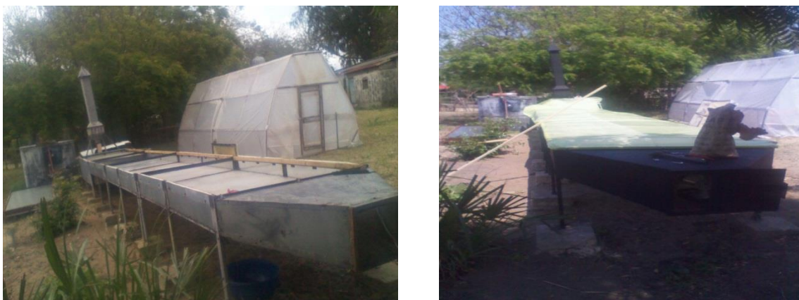
Figure 2.3: The collector roof of the dryer: Before (a) and after (b) roof installation
