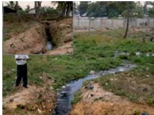
Figure 4: Uncontrolled sewage disposal into a wetland in Kisauni
